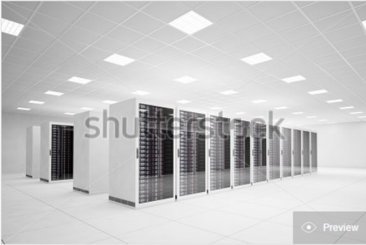
Figure 4-30: Data center cabinets and aisles. Image ID:156554486
